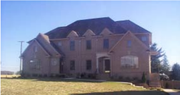
Example of Affordable Dwelling Units for two or more families that mimic single family detached housing (“Great House”)
